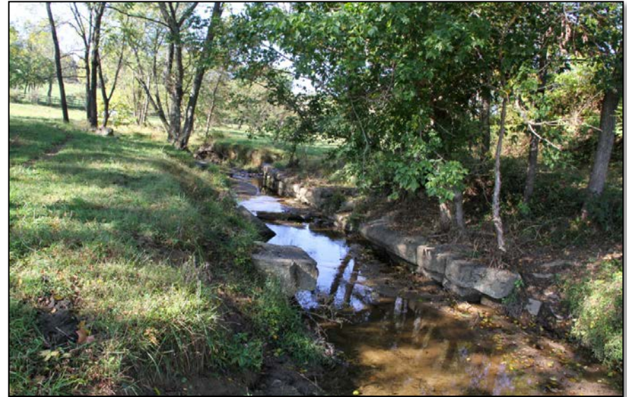
One of the culverts still visible today near the Foundry Rd and Taylor Rd intersection.
